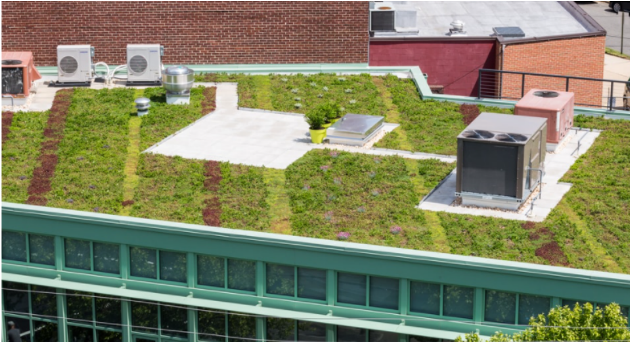
Figure 2: Example of a vegetated roof.
